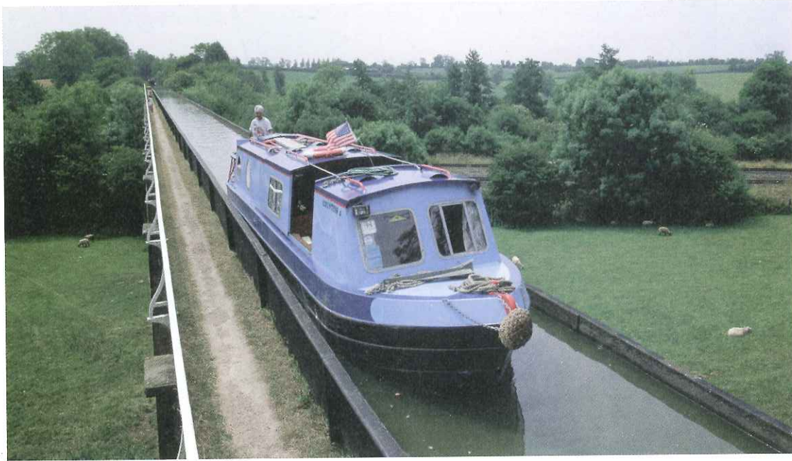
Figure 5–9 Today, the canals are used for pleasure boating. An aqueduct carries this canal over a valley.
